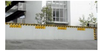
Tide protection gate
